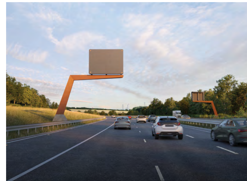
National Highways Gantries. The inclined upright permits maintenance access without safety caging.
