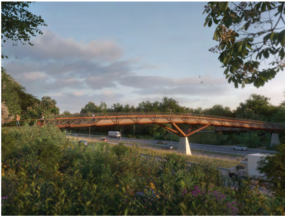
Salvaged Steel Footbridge
