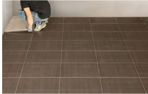
2. Install the first element, placing it perpendicular with the adjacent walls.
