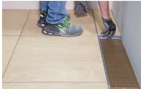
8. Fill any gaps between the elements and the wall with silicone.
