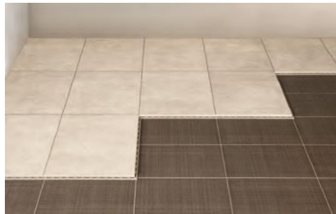
2. Install the first element, placing it perpendicular with the adjacent walls.
