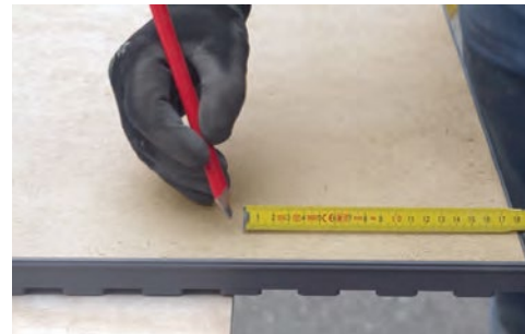
5. When done, cut elements to size around the edges if necessary.
