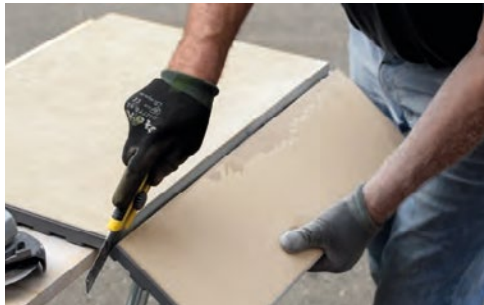
7. Cutting of the PUR using a jigsaw with laminate blade.
