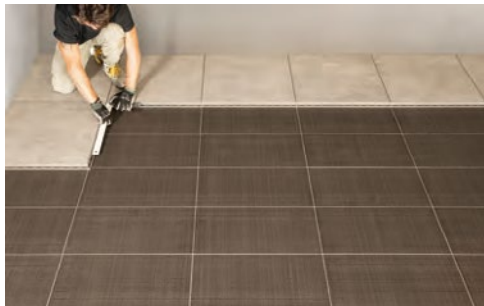
4. When the first row is complete, start again from the beginning, always ensuring that the elements are perpendicular.
