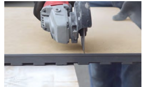
6. Elements can be cut with a tile cutter or angle-grinder.
