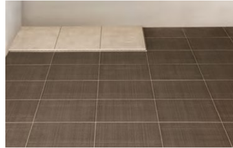
3. Continue installing, interlocking all elements on the right side, until the space is full.
