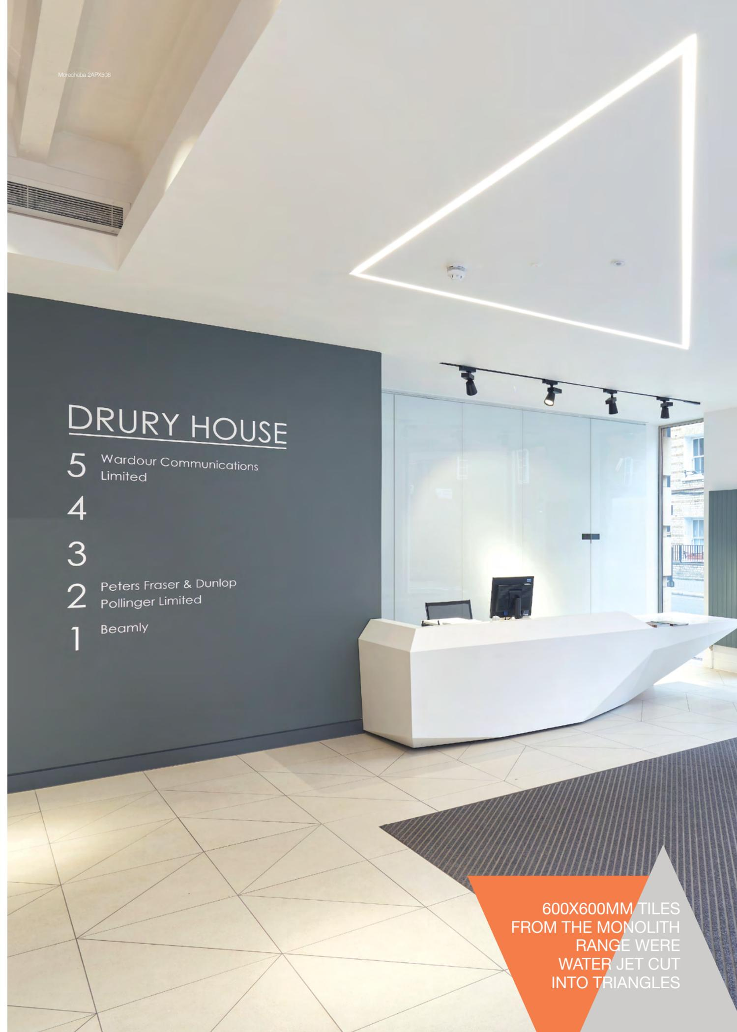
600X600MM TILES FROM THE MONOLITH RANGE WERE WATER JET CUT INTO TRIANGLES
